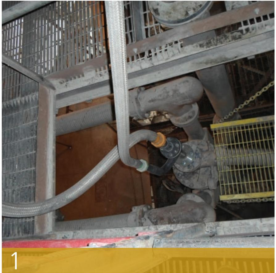
1. VISTA IN PIANTA DEL BRUCIATORE GRECO DEL CALCINATORE CON I RACCORDI FLESSIBILI PER L'ARIA E IL COMBUSTIBILE LIQUIDO DA RIFIUTI / PLAN VIEW OF CALCINER GRECO BURNER PIPE WITH AIR AND LIQUID WASTE FUEL FLEX HOSE CONNECTIONS
